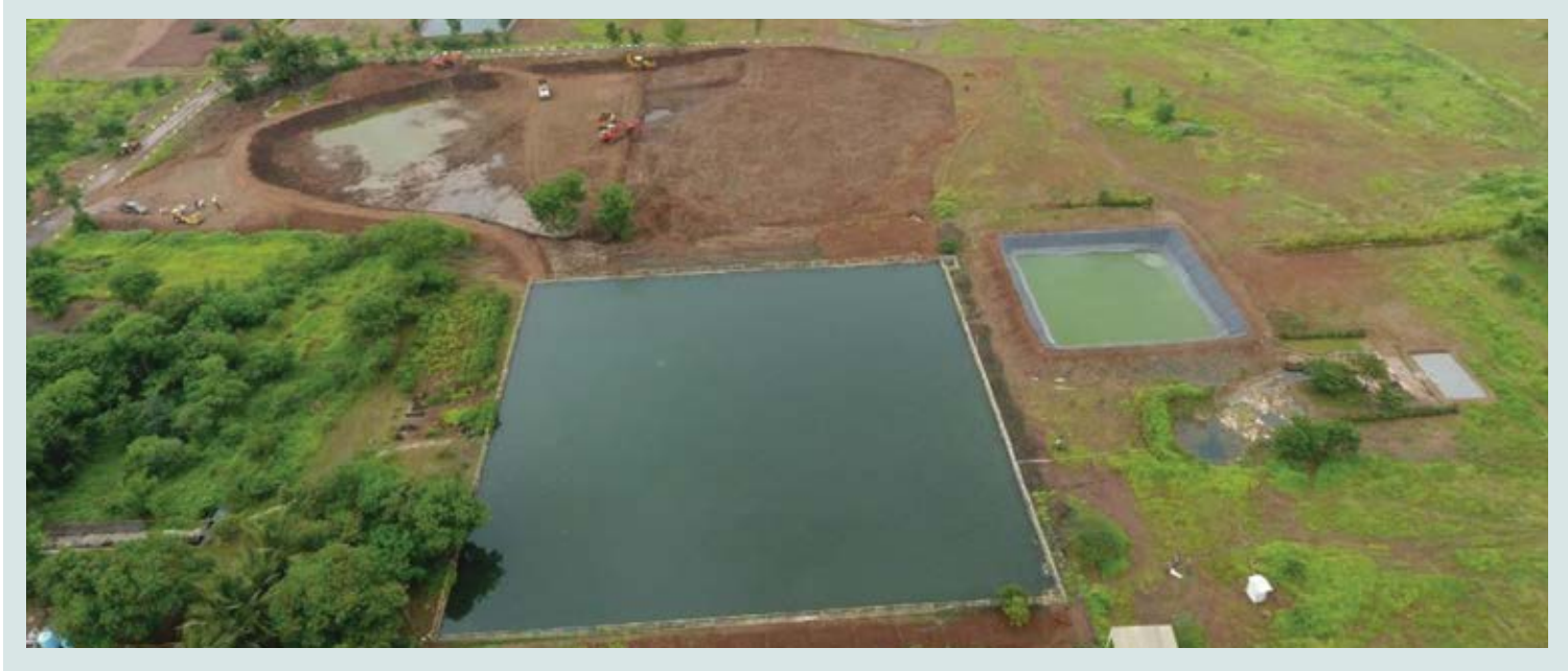
Rainwater harvesting pond
