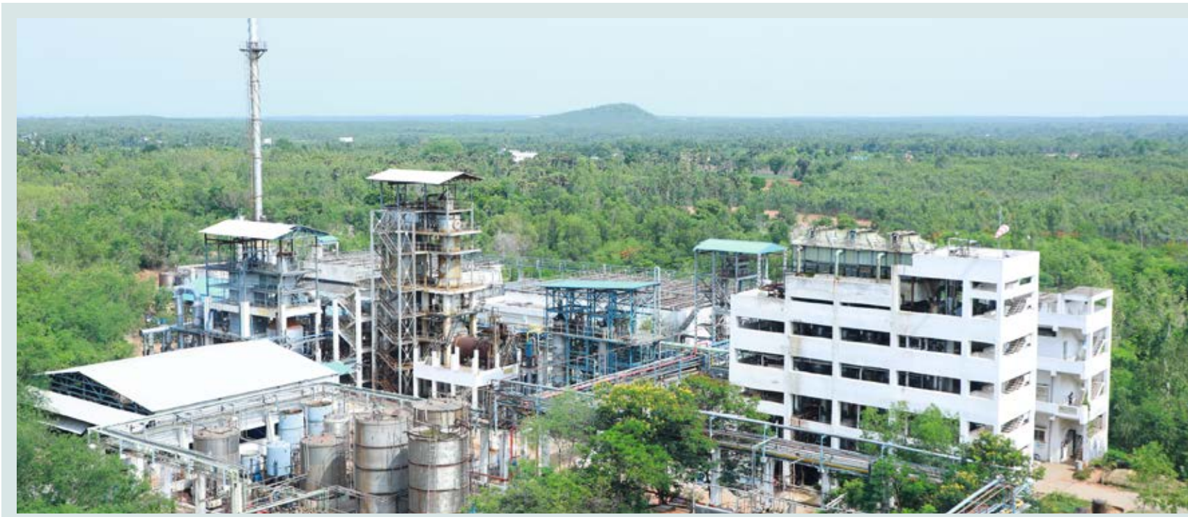
NAFL - Zero Liquid Discharge facility
