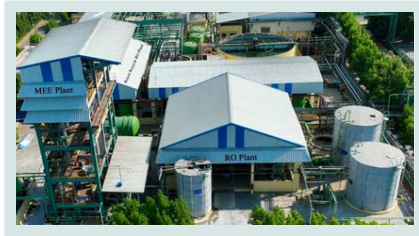
Zero Liquid Discharge Unit
