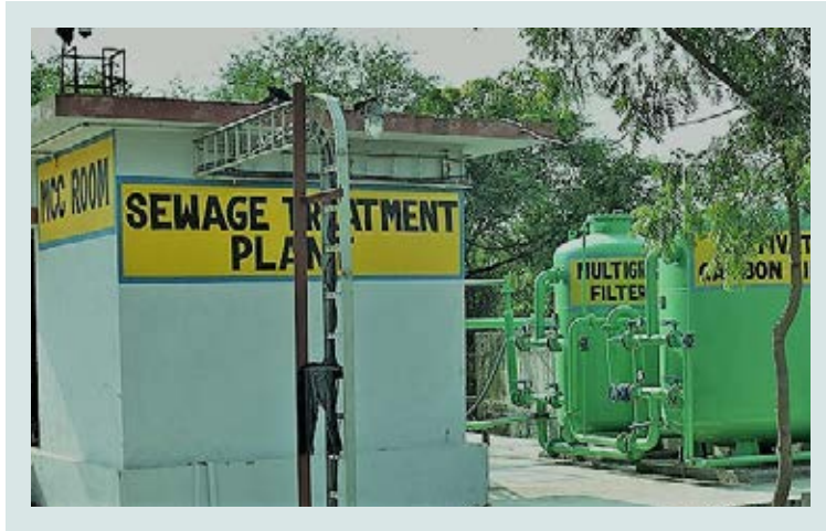
Sewage Treatment Plant
