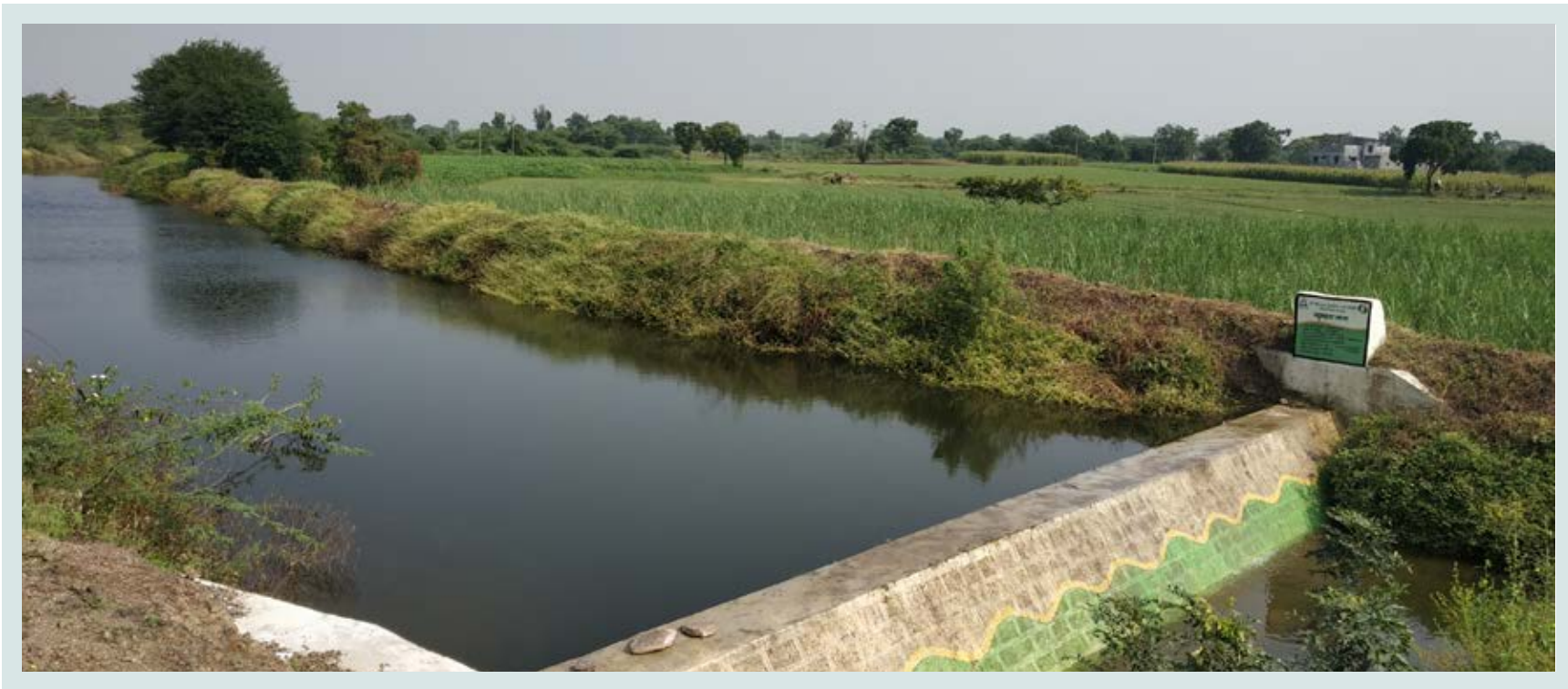
Water harvesting structure (check dam), Uralgaon Village, Shirur block, Pune district
