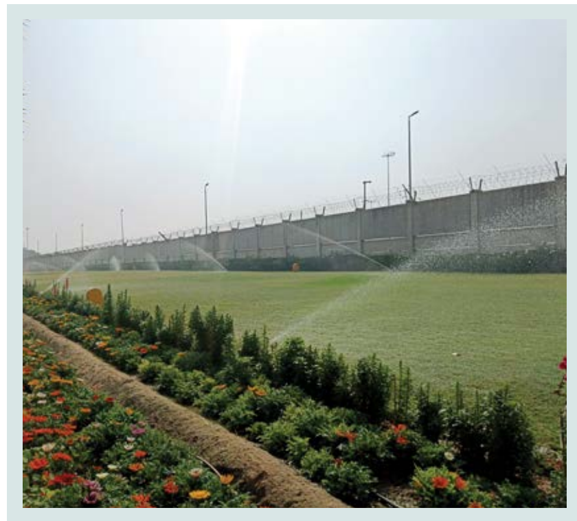
Advanced and efficient automated drippers, sprinklers system.
