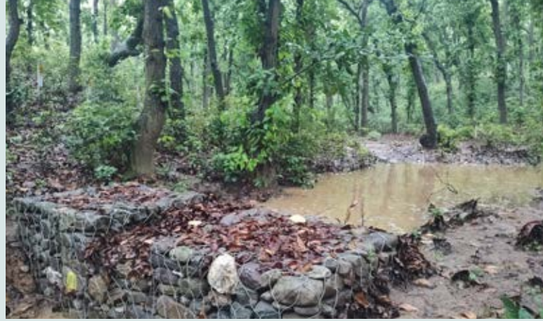
Gabion check dam, Naurangabaad reserve forest area, Paonta Sahib
