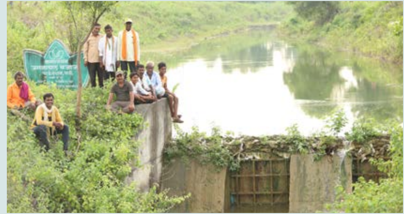
Check dam, Wardha, Maharashtra
