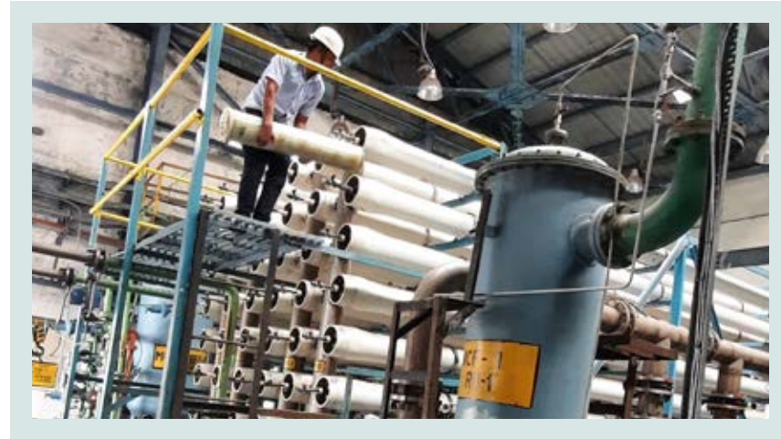
Membrane unloading for inspection
