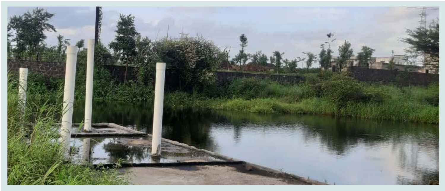
Ground water recharge pit
