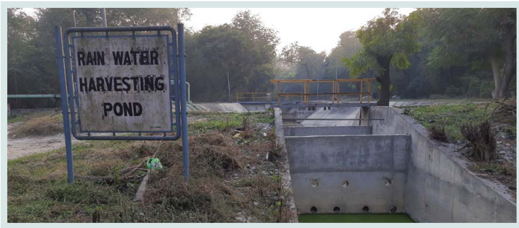
Plant catchment area project with rainwater harvesting potential of 128,500m 3 /annum
