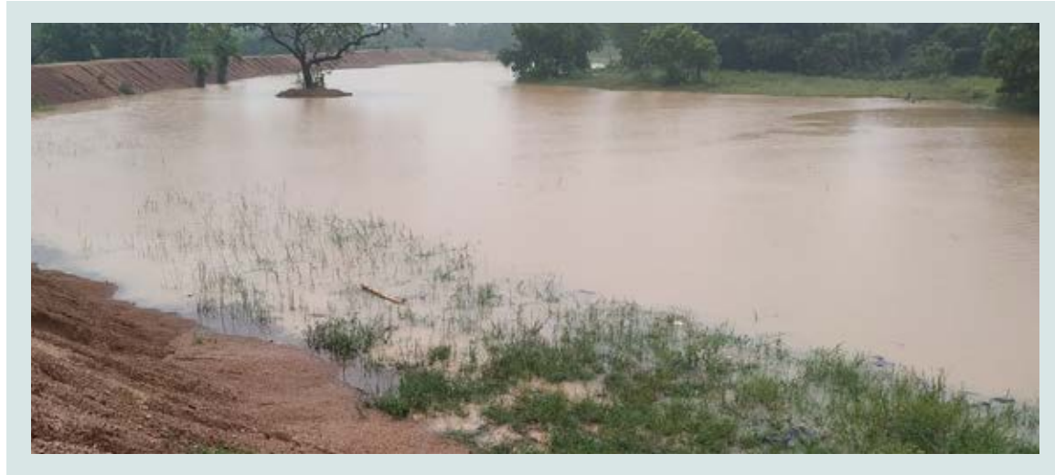
Restored Minor Irrigation Tank, Pattikadu
