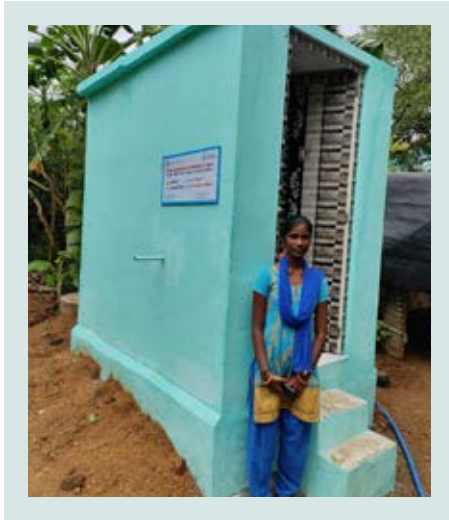
Toilet facility built for 5 BPL families with girl children, Pattikadu
