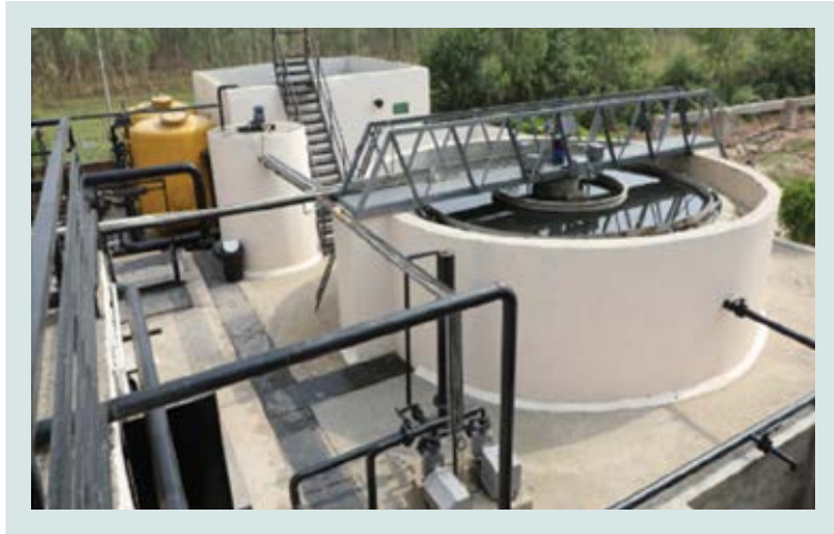
Sewage Treatment Plant
