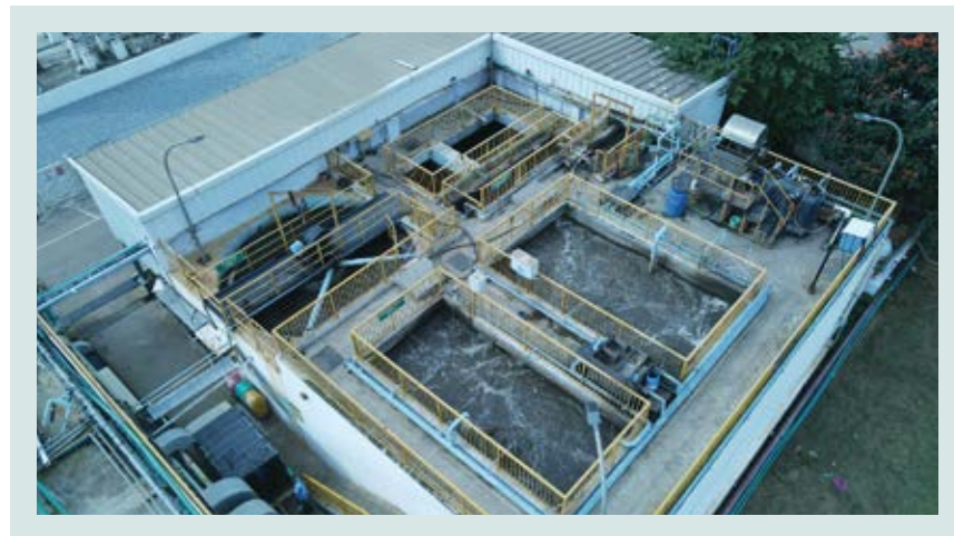
Aerial view of STP
