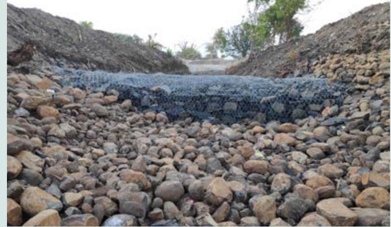
Gabion bandhara, Wadmurambi, Latur
