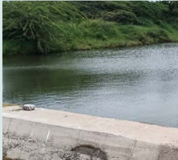
Check dam, Jakhar
