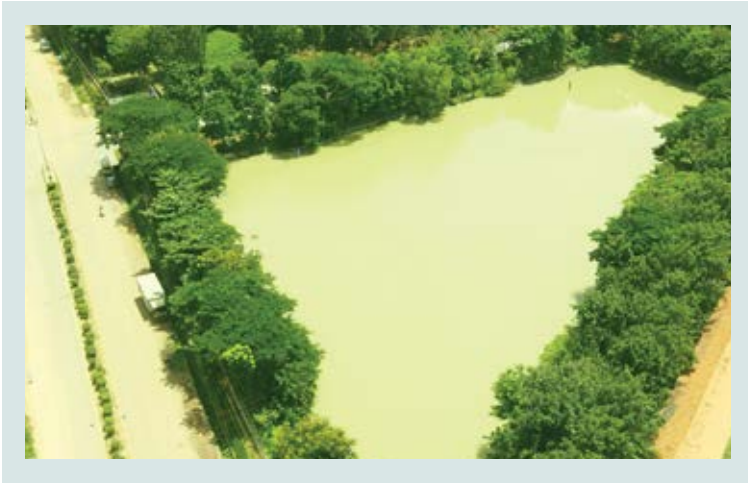
Open water tank-23000m 3
