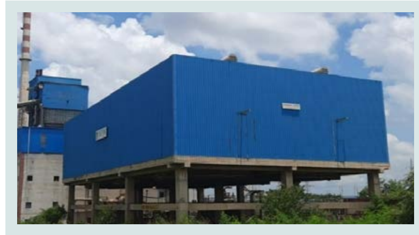
Waste Heat Recovery System (WHRS)
