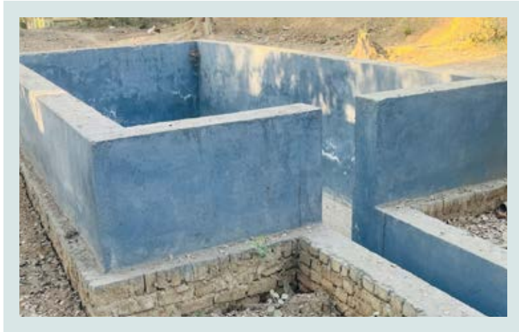
Recharge Injection Well
