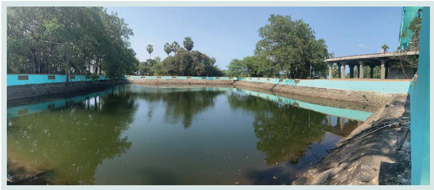
Renovated drinking water pond, Pattikadu
