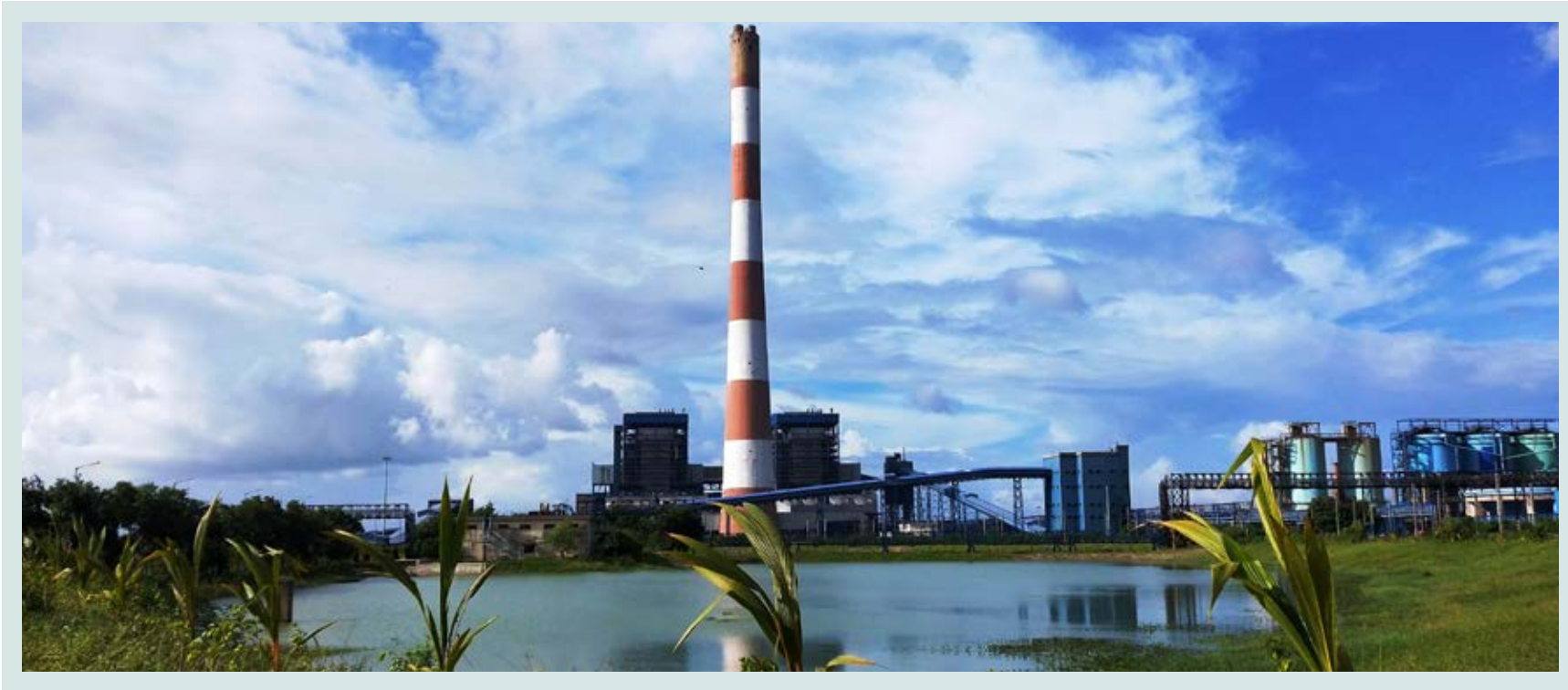
Rainwater harvesting pond with a capacity of 89,000m 3 has been created within the plant premises
