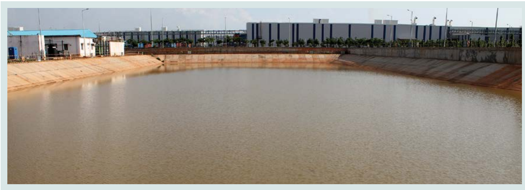
Storm water collection pond 27000m 3 capacity
