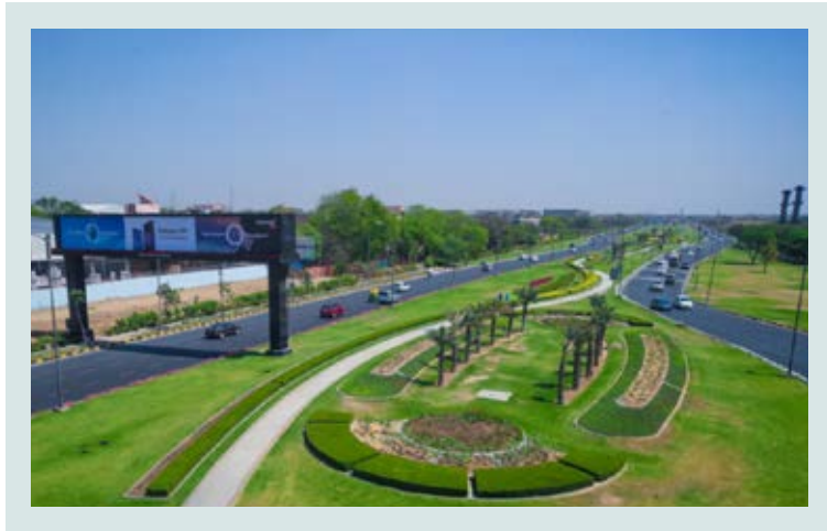
Green Corridor at IGI Airport- advanced microprocessor based smart irrigation system
