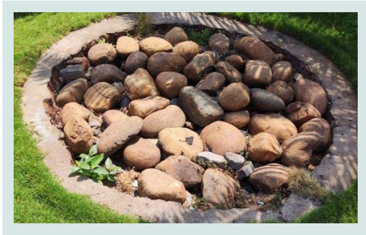
Rainwater harvesting system to recharge the ground water, G.Kuppuswami Memorial Hospital, Coimbatore
