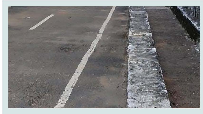
Trench Rainwater collection trench along plant periphery
