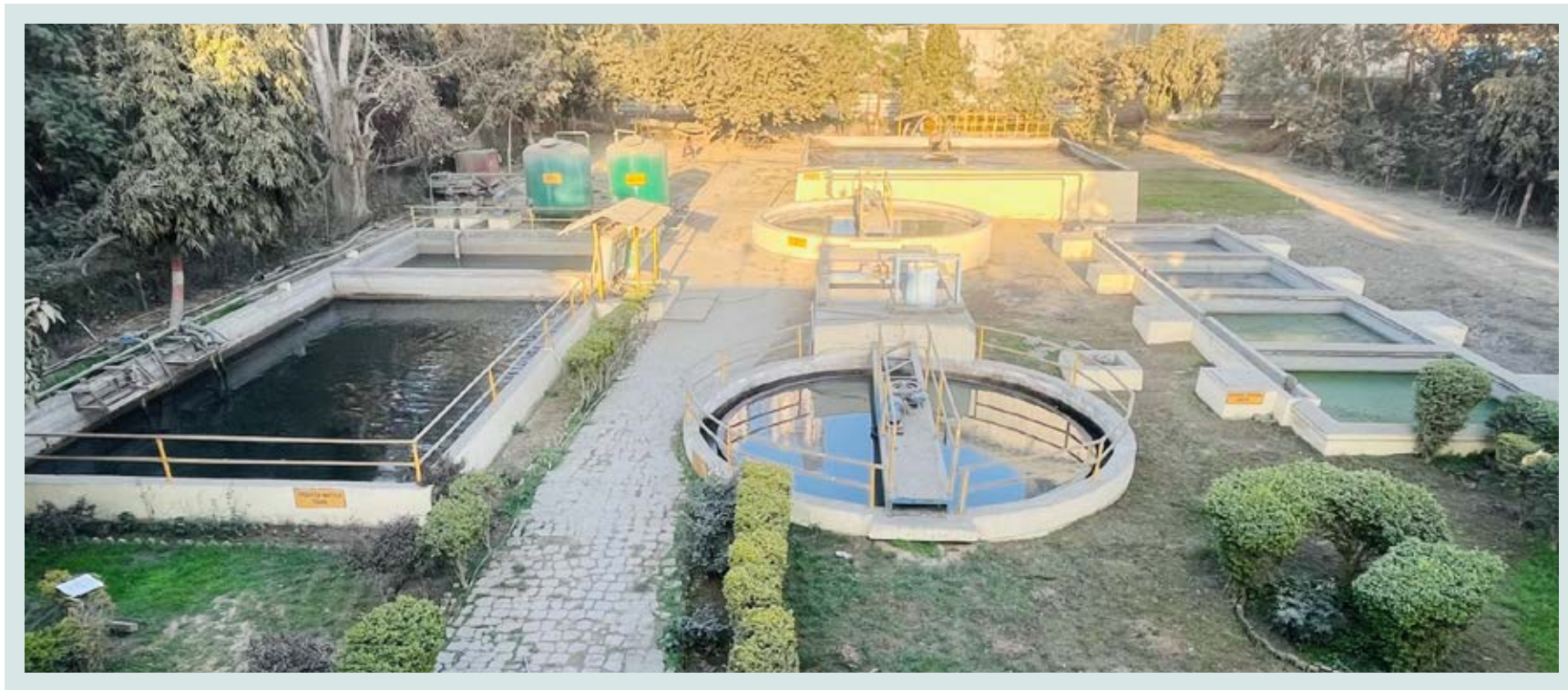
Sewage Treatment Plant
