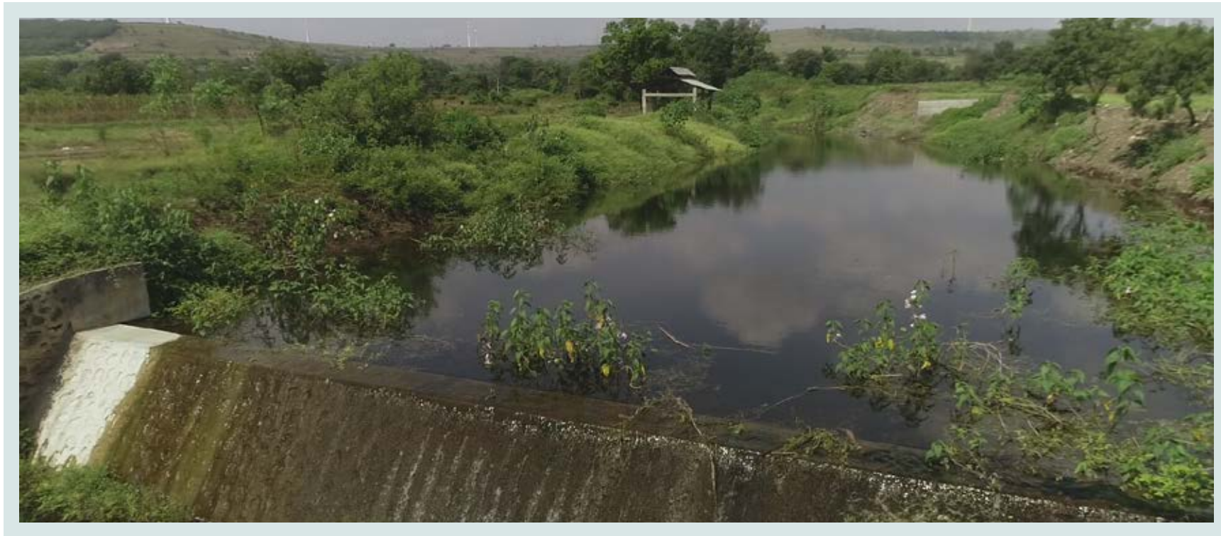
A cement nala bund to reduce water run off and increase water percolation
