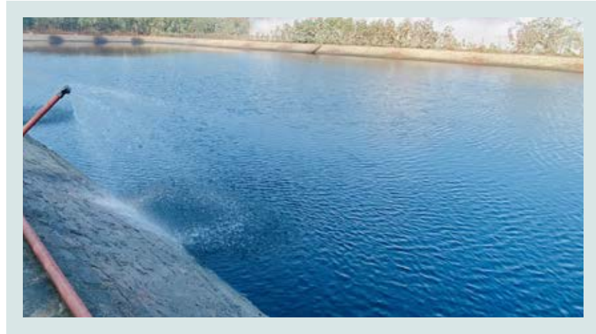
Lagoon - storage of reuse and recycled water to reduce borewell extraction
