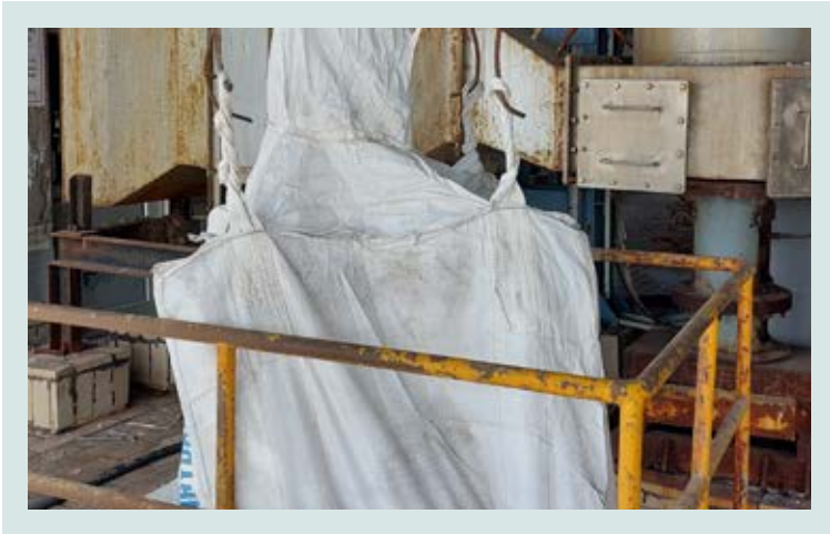
Sodium sulphate bagging system
